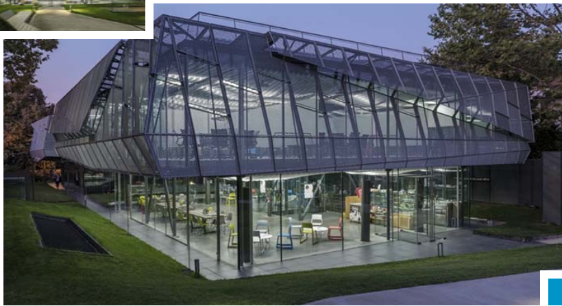
IYZIPARK OFFICE COMPLEX STRUCTURAL STEEL WORKS MANUFACTURING AND ERECTION ALTUNIZADE/ISTANBUL
