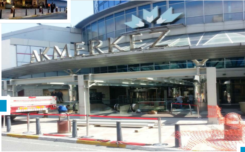
AK MERKEZ AVM ENTRY CANOPY MANUFACTURING AND INSTALLATION ETILER/ISTANBUL
