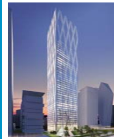
ISTANBUL TOWER 205 STRUCTURAL STEEL WORKS MANUFACTURING AND ERECTION LEVENT/ISTANBUL
