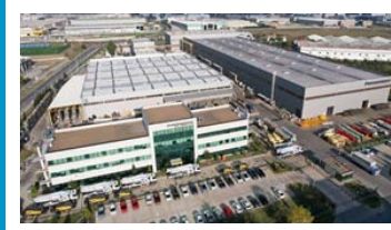
PUTZMEISTER CONCRETE PUMPS FACTORY CRANE BEAMS AND STRUCTURAL STEEL WORKS MANUFACTURING AND ERECTION CERKEZKOY/ISTANBUL
