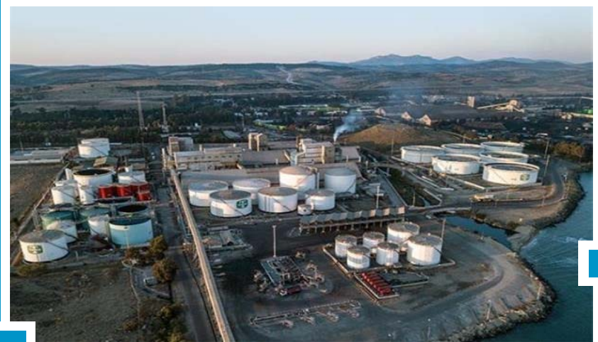
TOROS FERTILIZER AND CHEMICAL INDUSTRY A.S. PROJECT DESIGN AND APPLICATION OF 100.000 TONS CAPACITY STORAGE TANKS AND PUMP STATIONS CEYHAN/ADANA
