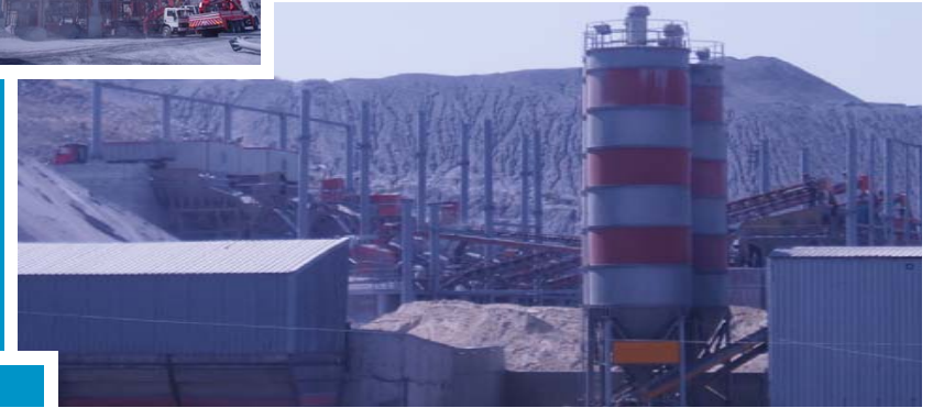
HAS BETON VARIOUS STEEL CONSTRUCTION MANUFACTURING AND INSTALLATION SULTANGAZI/ISTANBUL
