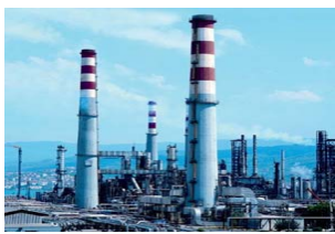
IPRAS 2. ENLARGING PROCESS CONTROL AND TESTING WORKS YARIMCA/KOCAELI
