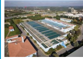
ISKI KAGITHANE DRINKING WATER TREATMENT PLANTS STEEL CONSTRUCTION MANUFACTURING AND INSTALLATION KAGITHANE/ISTANBUL
