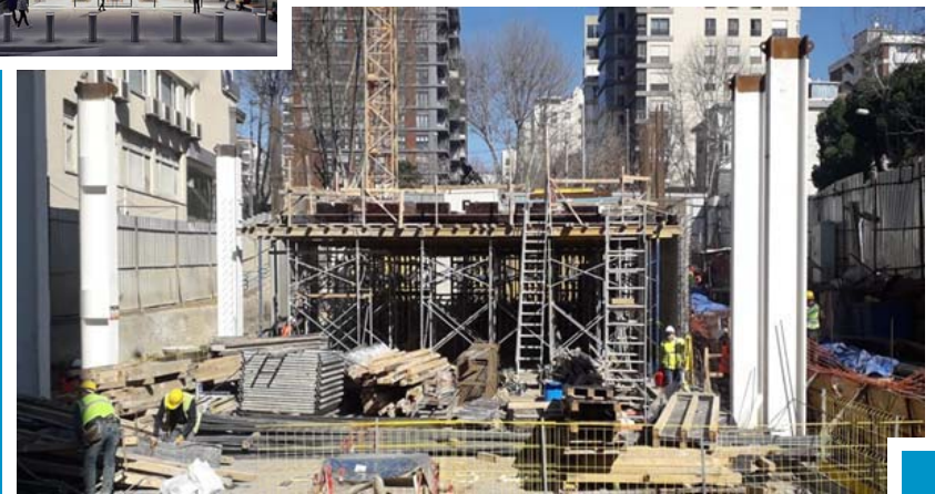
APPLE STORE BAGHDAD STREET STRUCTURAL STEEL WORKS MANUFACTURING AND ERECTION KADIKOY/ISTANBUL
