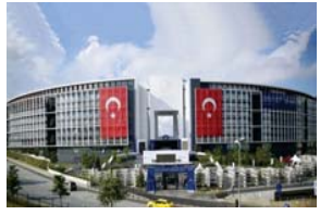
MEDIPOL UNIVERSITY KAVACIK CAMPUS STRUCTURAL STEEL WORKS MANUFACTURING AND ERECTION BEYKOZ/ISTANBUL
