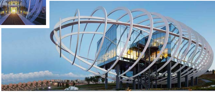
TEMAPARK SALES AND REPRESENTATION OFFICE CONSTRUCTION KUCUKCEKMECE/ISTANBUL
