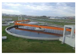
ISKI SELIMPASA WASTEWATER TREATMENT PLANTS STEEL CONSTRUCTION MANUFACTURING AND ERECTION SILIVRI/ISTANBUL
